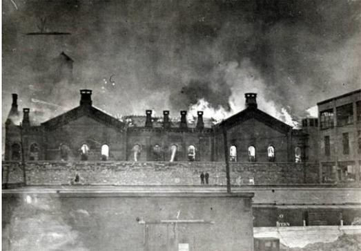
5. New London School, New London, TX: An undetected natural gas leak was ignited by an electric sander on March 18, 1937, causing an explosion and fire that killed approximately 300 people.
